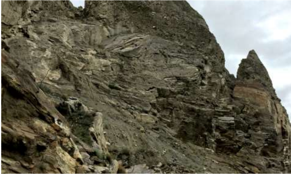
Photo 4-69 Development of Longitudinal Joints in Rock along KKH.
