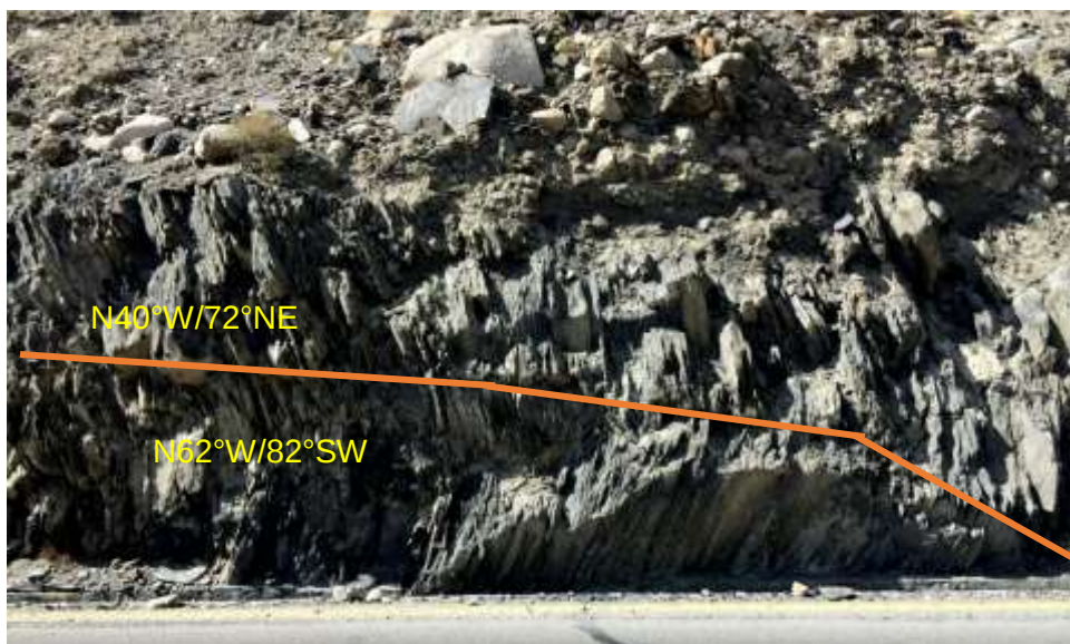
Photo 4-13 Change of Dip along Shear Joint.
