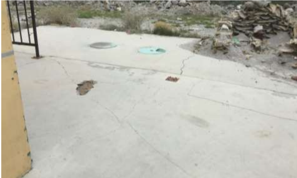
Photo 4-55 View of Recently Generated Joints between Tunnel-2 & 3.
