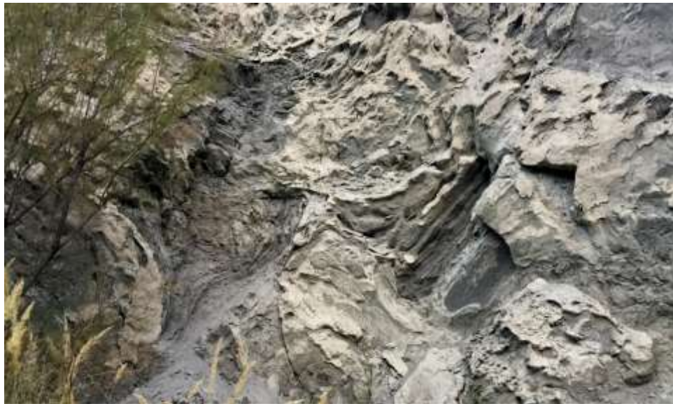
Photo 4-39 Sheared and Smeared Clayey Silt at Sarat Village.
