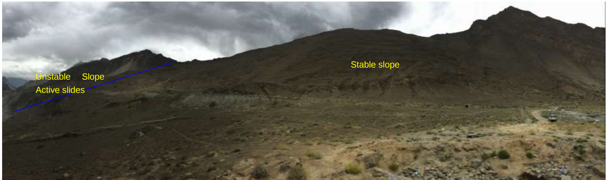
Photo 4-63 Panoramic View of Slope in front of Salmanabad and Ahmadabad Village
