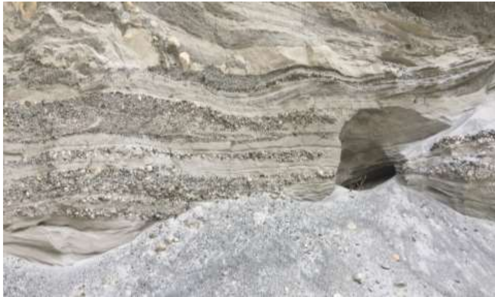
Photo 4-23 Inward Inclination(curvature) of RBGM and Sand Beds.
