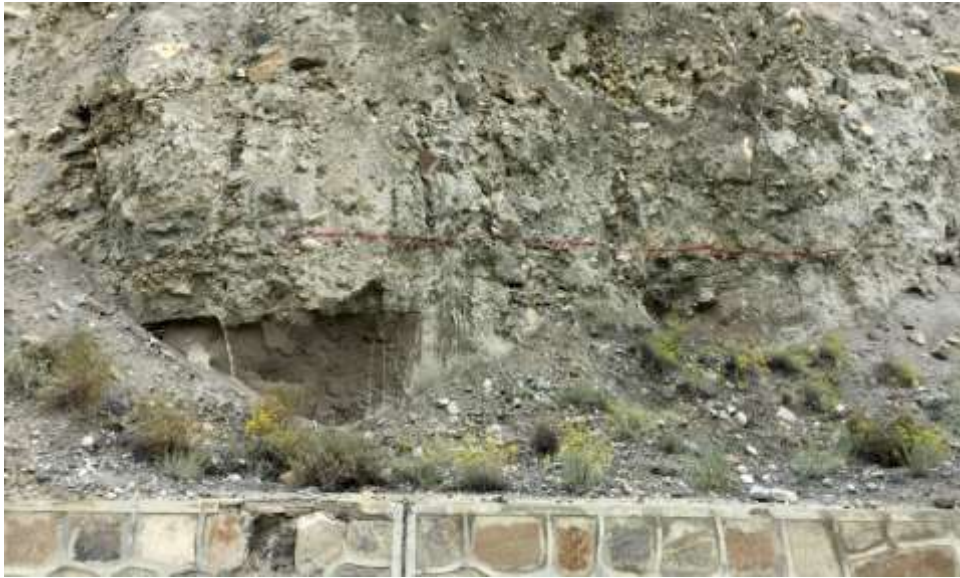
Photo 4-67 Inclination in ABGM and Clayey Silt Bed along KKH.
