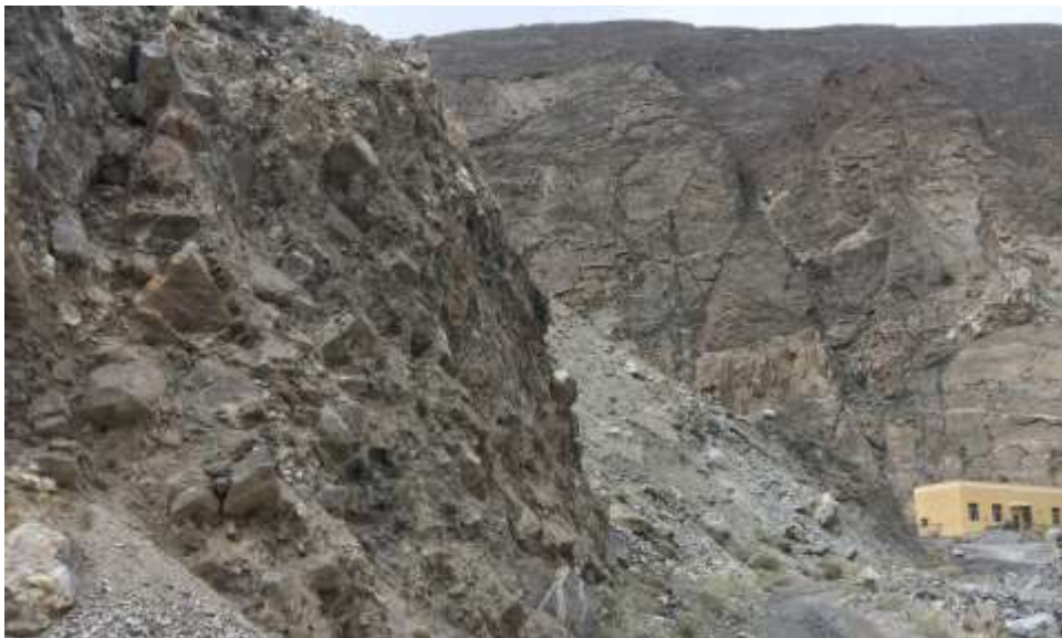
Photo 4-56 View of Fault Breccia between Tunnel-2 & 3.
